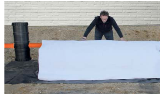
Cover tunnel with GT-300
